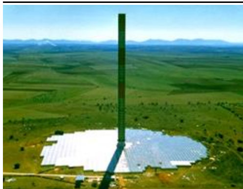
Figure 74: Photovoltaic Solar Tower
