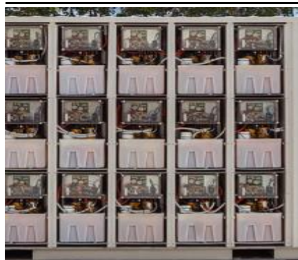
Figure 75: Flow Battery Assembly
